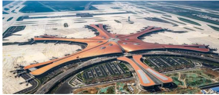
Fig. 1 – Daxing International Airport
